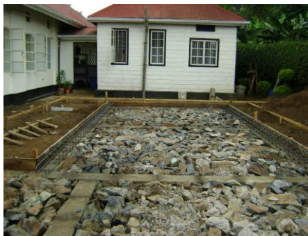
Figure: Foundation of the new building
